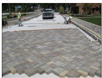
At work on installing the pervious pavers.
